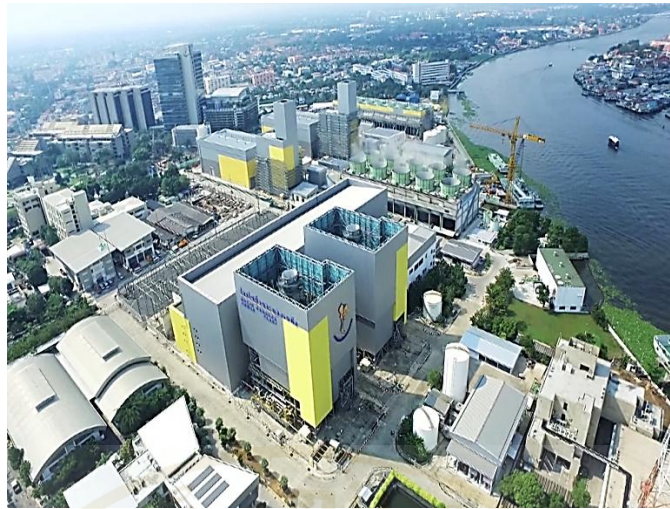
Figure 1.12 Location of North Bangkok Combined Cycle Power Plant Unit 1
