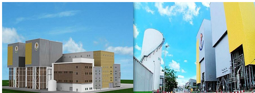
Figure 1.9 North Bangkok Power Plant Combined Cycle Unit 1
