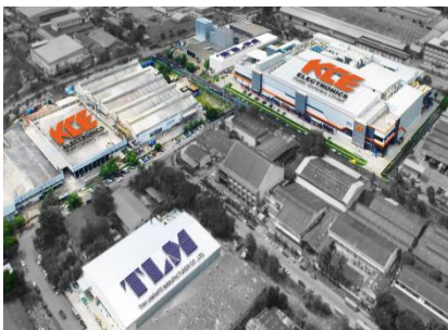
Figure 2.1 KCE manufacturing in Lat Krabang
