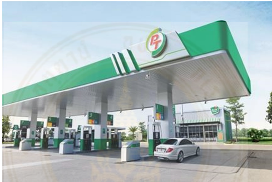
Figure 2.3 A PT gas station
